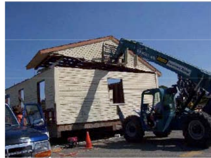
Figure 2.2 Roof is removed to ground level where it is safer and faster to deconstruct
