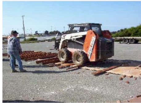
Figure 2.7 Removing studs from sheathing using the Drive-By method
