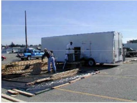
Figure 2.11 Trailer is parked at the deconstruction site, it is negatively pressurized to contain lead paint dust.
