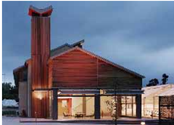
Figure 4.1 Global Ecology Research Center - Steel Frame
