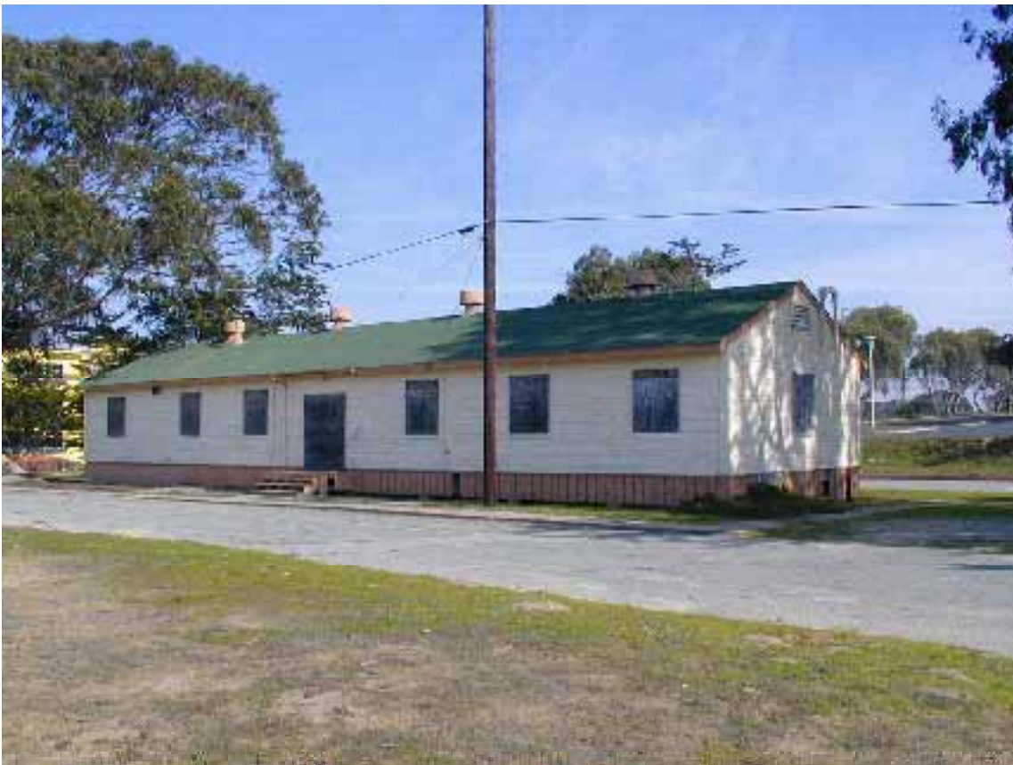
Figure 2.1 Typical Fort Ord Barracks building to be deconstructed, part of the “urban forest” that is being harvested for new construction projects
