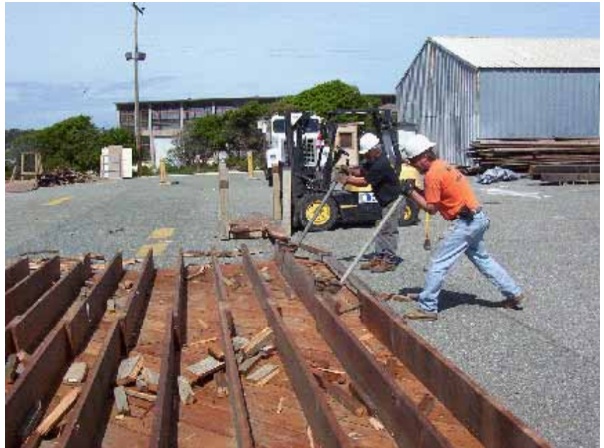
Figure 2.6 Removing joists from sheathing with custom made pry bars
